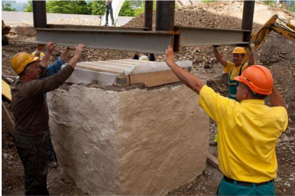
Fig. 9: With the help of the construction team and their machinery the specially manufactured steel frame is placed over the block.
