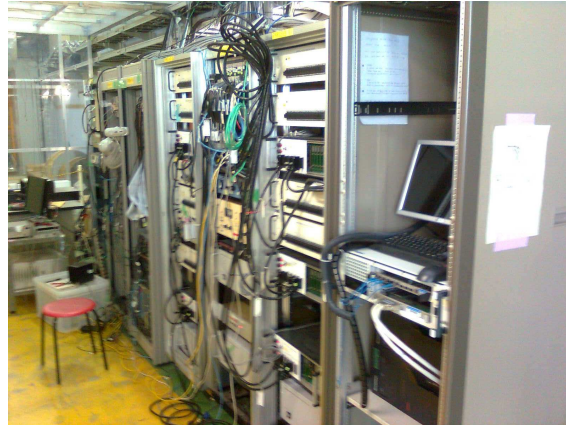
Figure 3.25: The Multi-OTR area in the so-called “eel’s bedroom” where the controllers and the host PC are located.
