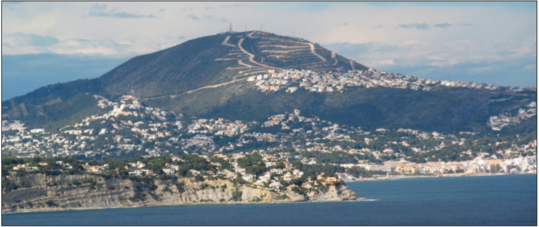
Fig. 6 – Discontinuous urban fabric in Benissa, Teulada and Benitatxell (northern Costa Blanca). Near the top of the hill we can see an urbanized area where the planned houses have never been started in fact because of the sudden Spanish housing bubble collapse. Now it spoils the landscape to no avail. Source: Antoni M. Bernat (2012)
