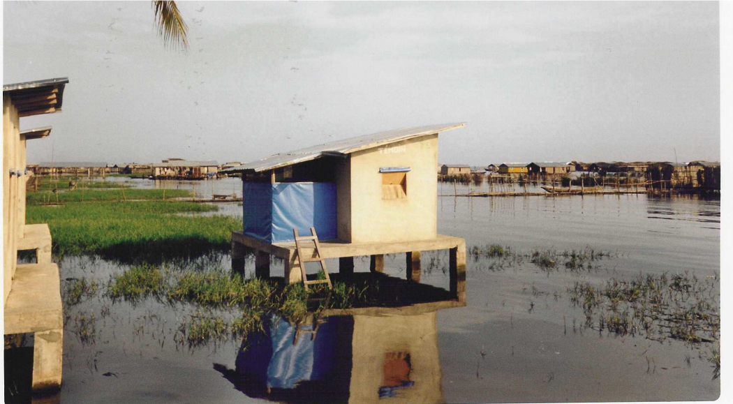
Figure 6: View of a WHOPE Phase II experimental hut at Ladj
