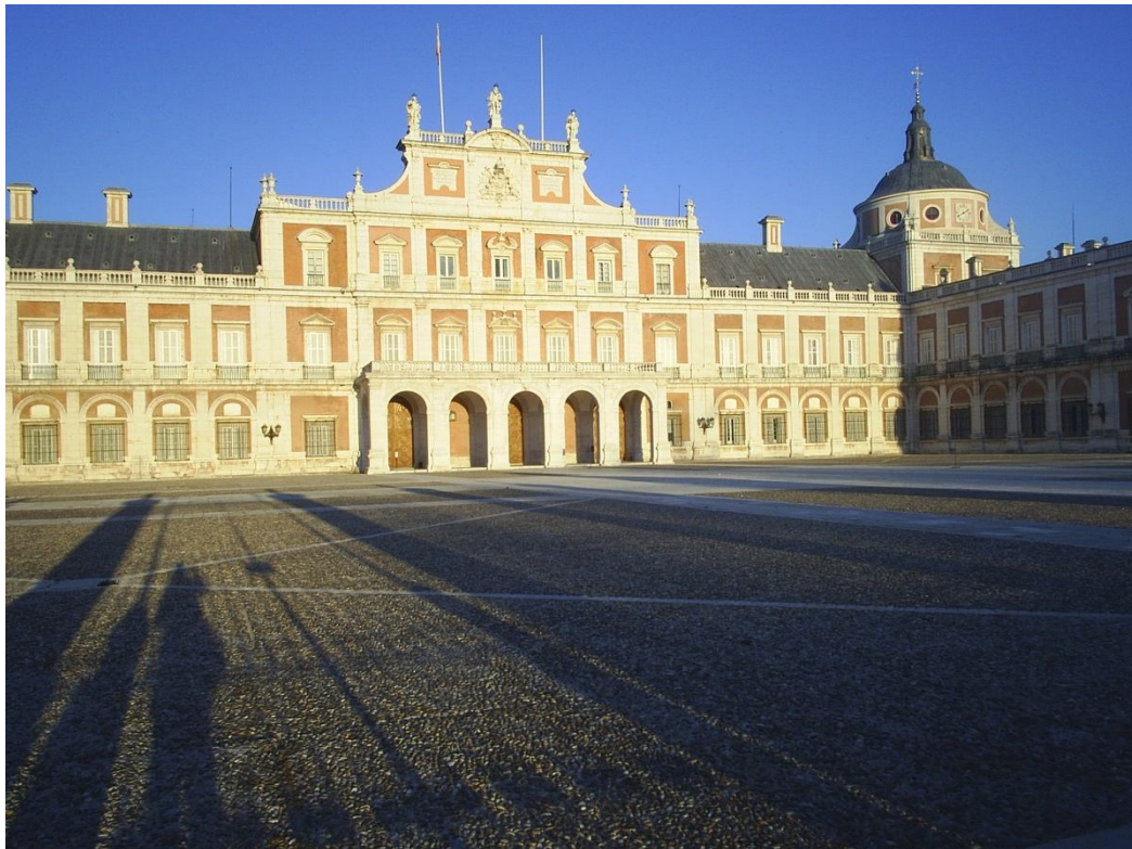
Fig. 226: Façade of the Royal Palace of Aranjuez
