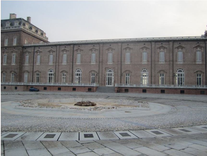
Fig. 109: Galleria Grande seen from the North
