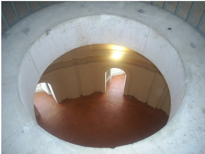
Fig. 222: Royal Palace of Aranjuez, interior southern tower
