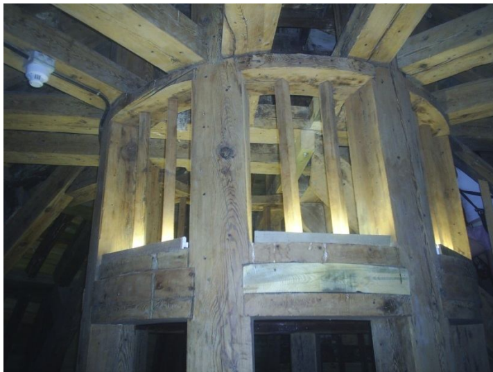
Fig. 256: Royal Palace of Aranjuez, southern tower, view of the central cylinder of the spire
