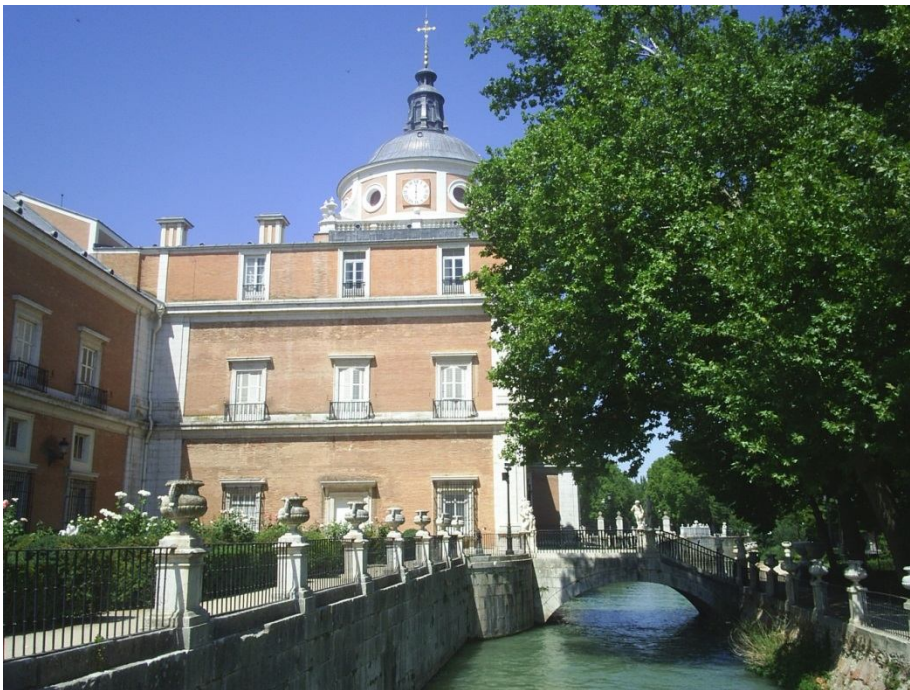
Fig. 237: Queen's garden with adjacent bridge
