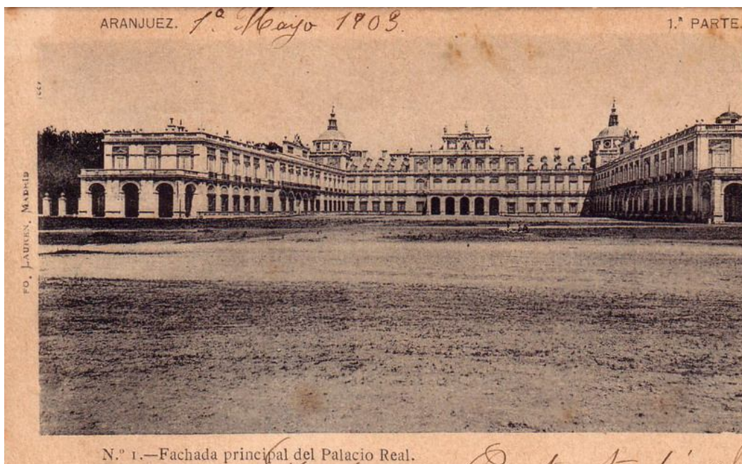
Fig. 195: Aranjuez, Main façade of the Royal Palace, May 1903
