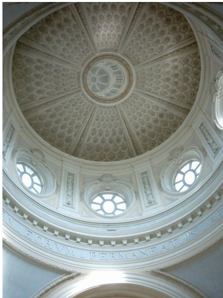
Fig. 50: Roof of the chapel of St. Uberto
