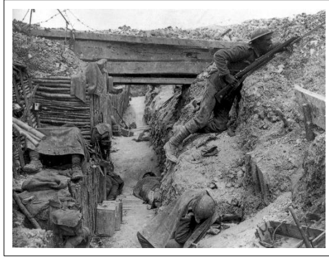
Fig. 7. In the trench.
