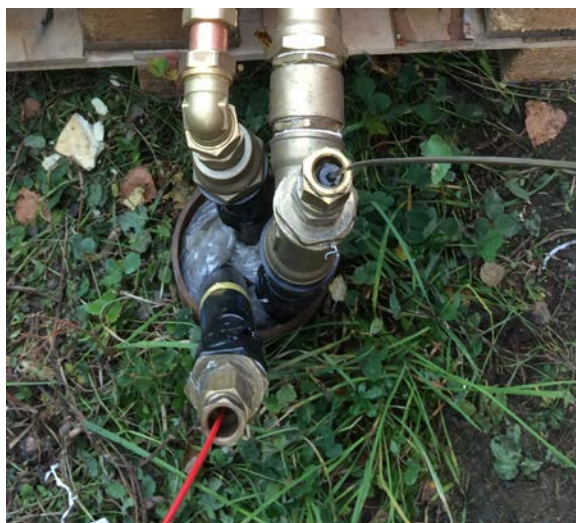
Fig. 15. Fiber optics installed inside geothermal pipes (Vallentuna, Sweden).
