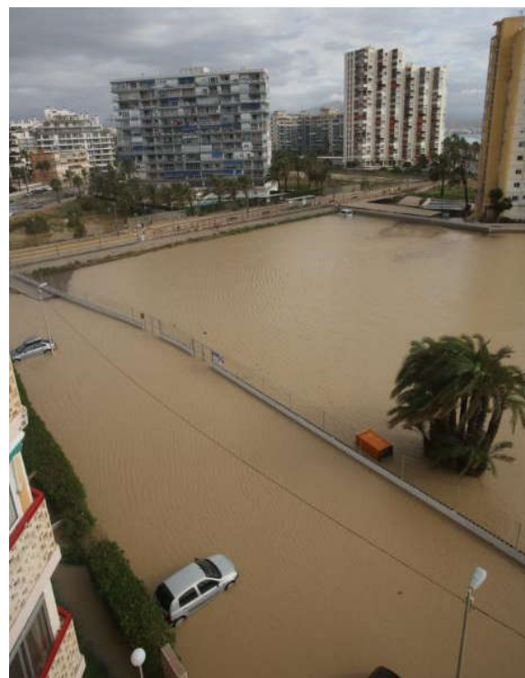
Figure 9. Old floodable area in San Juan Beach that has been urbanised since the 1960s. Note: episode of the 21 of August 2019. Source: [63].
