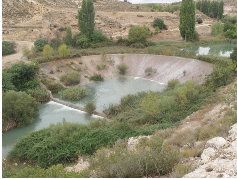
Figure 4. Presa de Moranchel, Mid-Júcar River.
