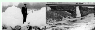
FIGURE 1. Foaming in sewage treatment and on rivers in the 1950s caused by non-biodegradable TPS (Düsseldorf).
