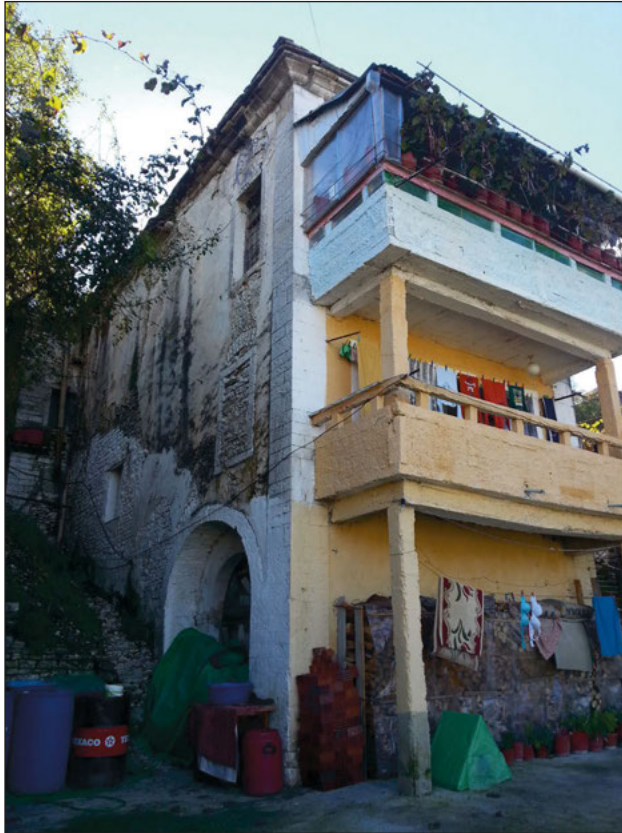
Figure 4. Informal extensions on historic buildings are common on most houses in the World Heritage area
