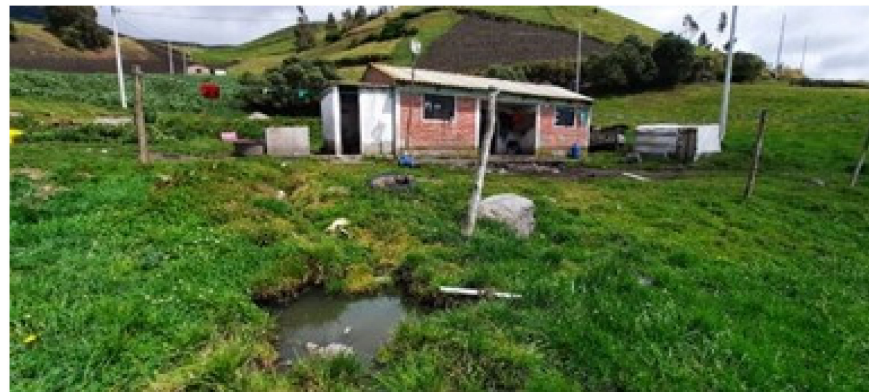
Figure 2. House with a leaky septic tank underground.
