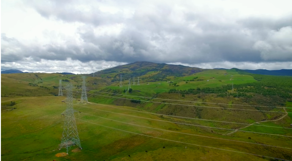
Figure A.19: Substation and transmission lines.
