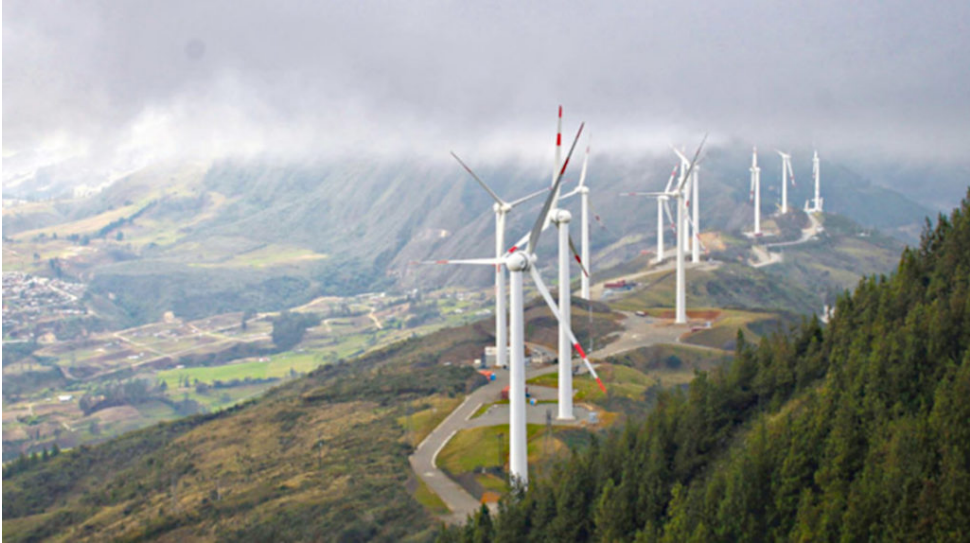
Figure 5.2: Panoramic view of Villonaco hill and Villonaco wind turbines.
