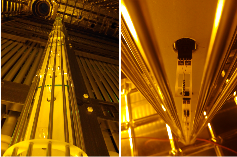
Figure 3.7: Static T-Gradient Monitor installed inside ProtoDUNE-SP cryostat.
